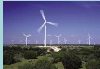
Courtesy of General Electric
